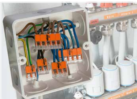
Wiring fine-stranded conductors in a junction box for in-floor heating.
