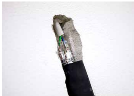
Connect the cable using the cable repair kit.
