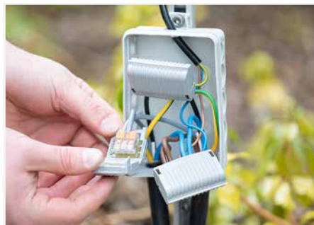
Connecting a bollard light
